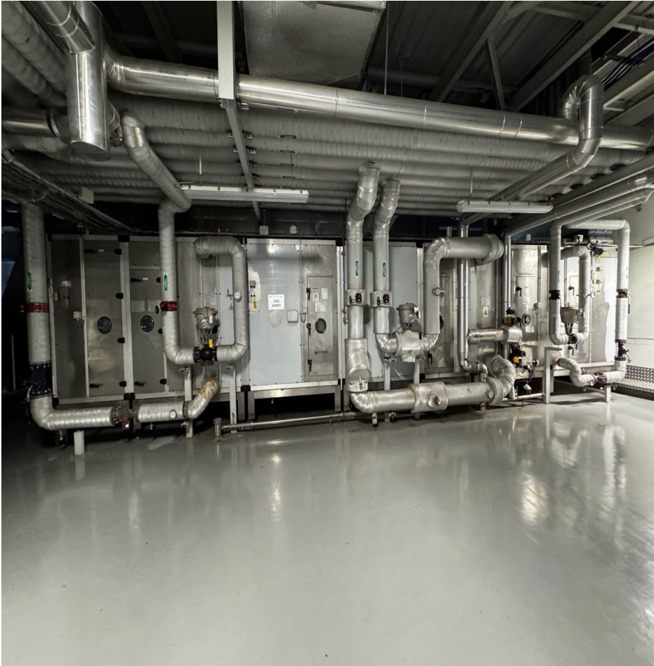
Fig 4.3 - UTA situate in penthouse
