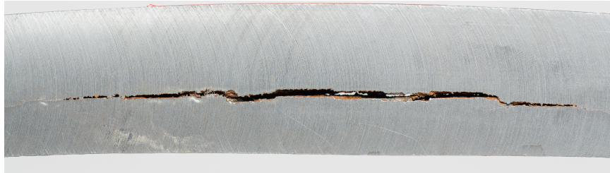
Figure 2.5: HE cracking. Photo by CEphoto, Uwe Aranas
